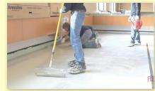
**Liquid Applied**Flexmar NextGen polyaspartics are poured and rolled onto the concrete flooring.
