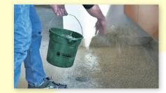
**Decorative**Vinyl chips are broadcast to rejection into the still-wet polyaspartic base coat.
