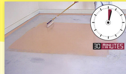
Base Coat Applied
