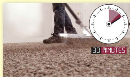
Excess Color Flakes Removed
