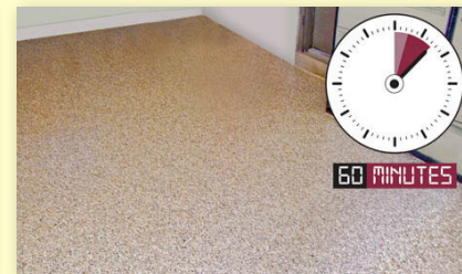
Allow Floor to Cure
