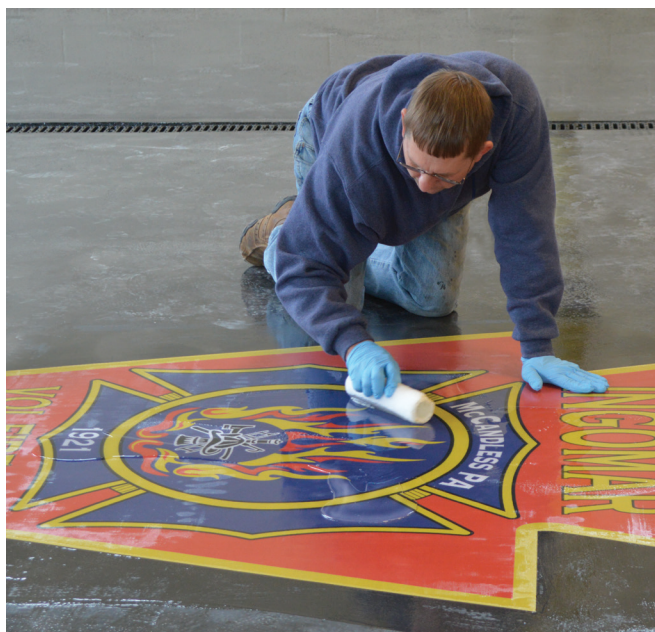
As a finishing touch, two logos, each sixty inches wide, were embedded in a final coat of FLEXMAR clear polyaspartic sealer.
