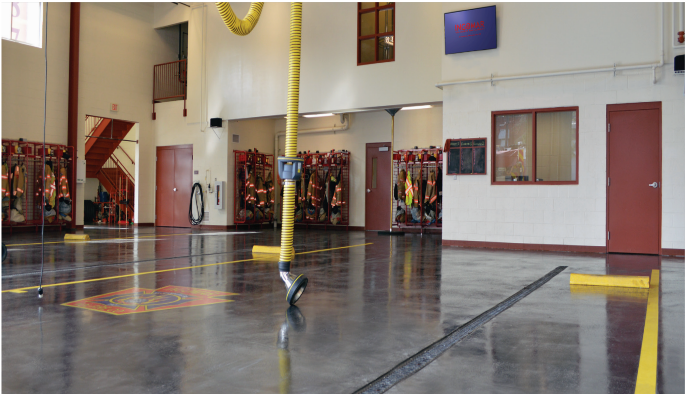
The FLEXMAR Variegate polyaspartic stain-sealer system was applied with minimal disruption to the fire company's normal operation.
