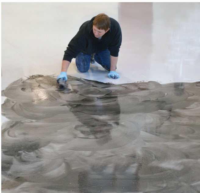
The FLEXMAR-qualified applicators at U-NEEK Concrete Coatings used a combination of a solid-color FLEXMAR polyaspartic coating and semi-transparent FLEXMAR Variegate polyaspartic stain-sealer to create a subtle look that resembled thick black smoke on the floor of the apparatus bays.
