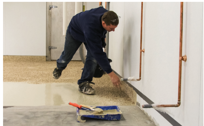
Applicators from U-NEEK Concrete Coatings applied a FLEXMAR 3-Coat High-Build Vinyl Chip polyaspartic coating system on the commercial kitchen floor. Coating application was completed in one day.
