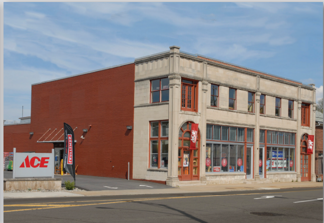
Renovated in 2011, the Ace Hardware in Greensburg, Pennsylvania was designed to elegantly incorporate older elements with modern fixtures.
