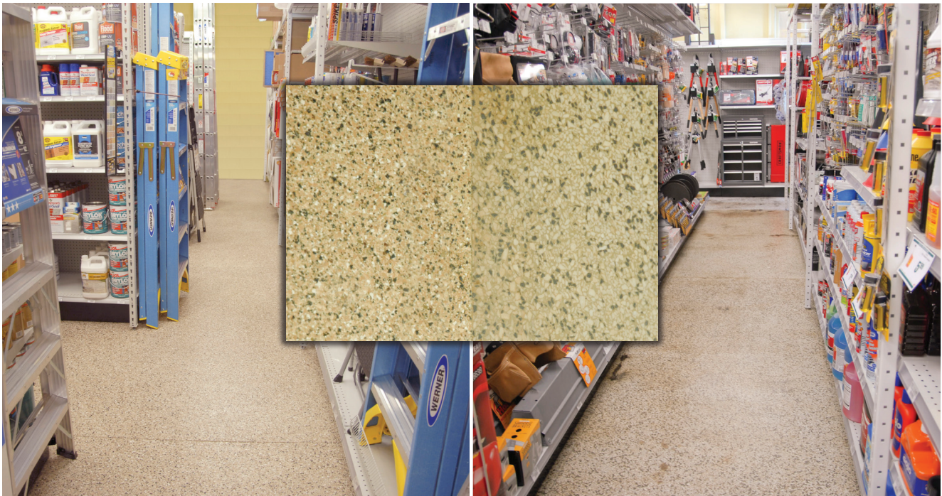
The FLEXMAR vinyl chip polyaspartic floor coating system, left, was chosen to closely match the original terrazzo floor, right, still present in the storefront.
