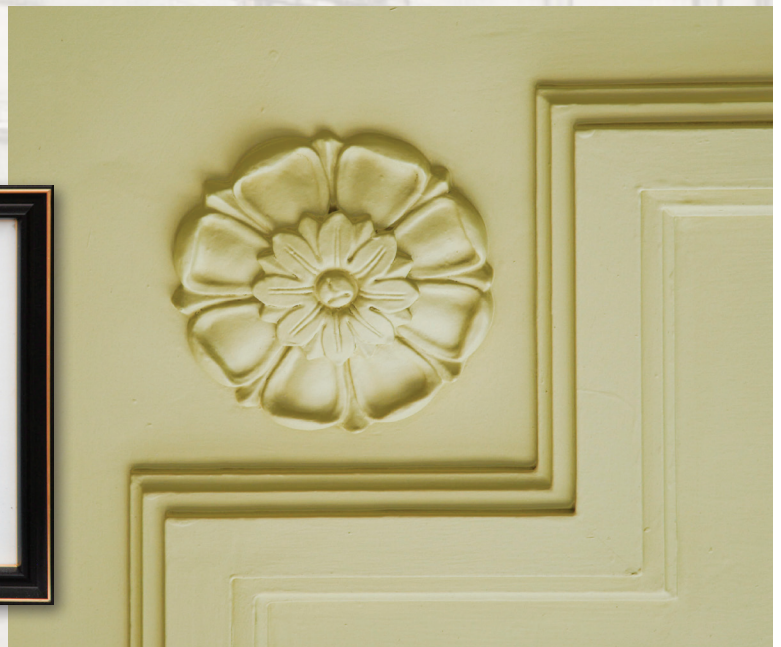
Demolition within the building during the restoration process revealed beautiful details to the interior's architecture.
