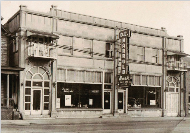
Built around 1926, the building that houses the Greensburg Ace Hardware served as a car dealership, repair garage, and equipment supply. (Photo courtesy of leeCALISTI architecture+design.)
