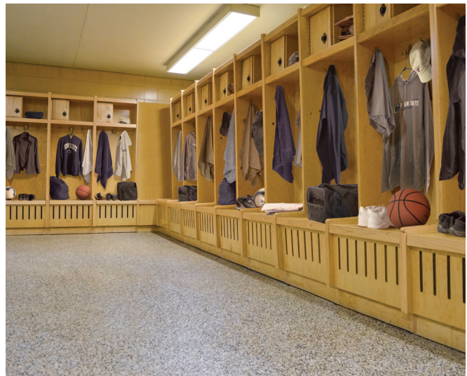
A FLEXMAR 3-Coat High-Build Vinyl Chip polyaspartic coating system was applied to the locker room floor as part of a complete renovation to the locker room facility, including painting and installing brand new lockers.
