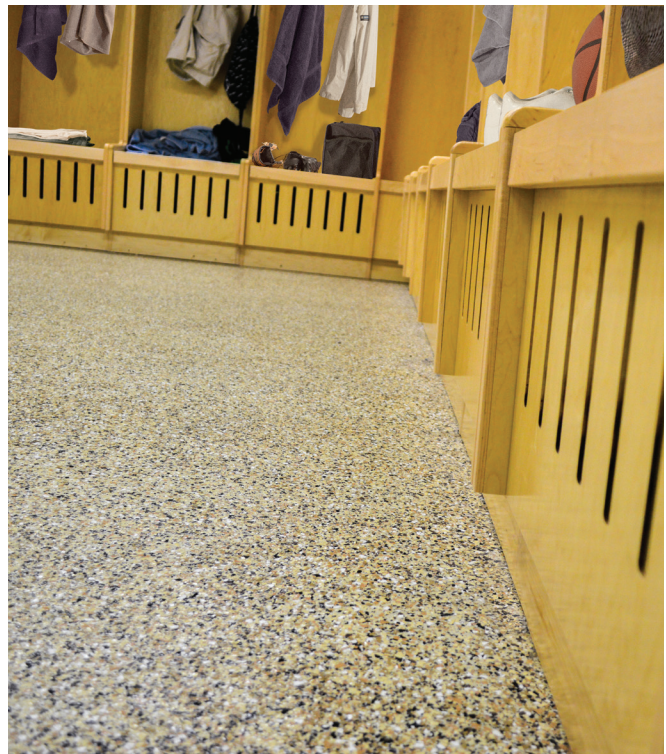
The new locker room facilities, with FLEXMAR vinyl chip polyaspartic coating system, enhances the athletic center's appearance and provides the look of excellence that Penn State student athletes expect.
